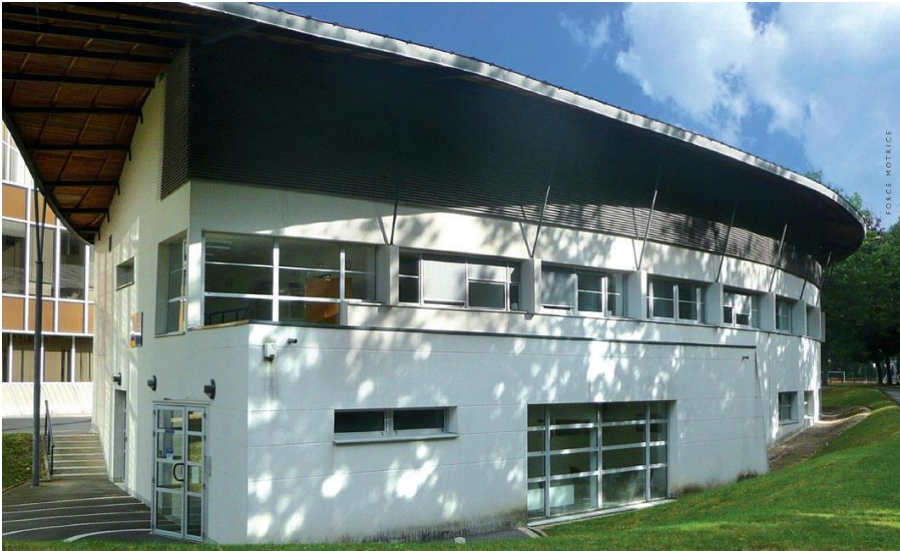
New SPS Pharma Services site in Orléans, France.
